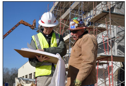
A barracks construction project at Fort Bragg, North Carolina.
