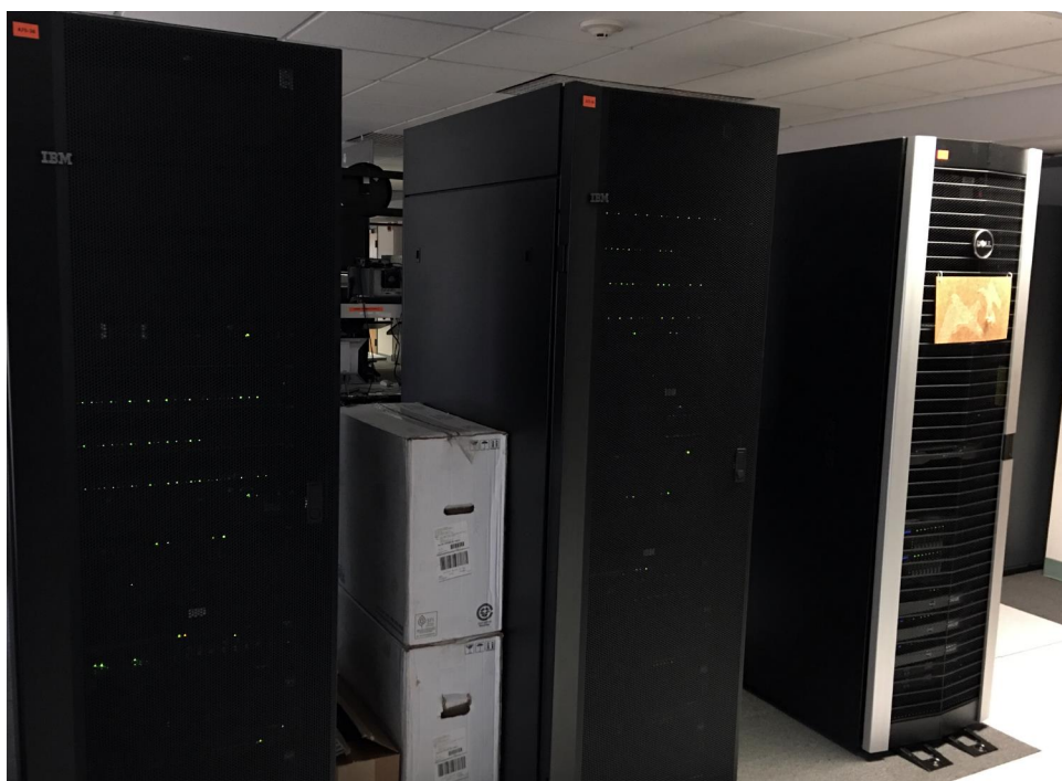
Figure 7: National Weather Service Telecommunication Gateway Server
