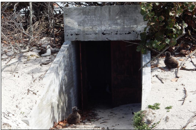
Figure 50: Underground Shelter (Property No. S956), Midway Atoll, Sand Island (April 15, 2015)
