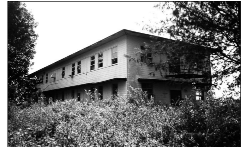
Source: U.S. Fish and Wildlife Service. | GAO-16-382 Marine Barracks (property number 579), 2007.
