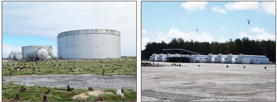
Figure 7: Photographs of Old Fuel System (Left) and New Fuel System (Right) on Midway Atoll, April 2015
