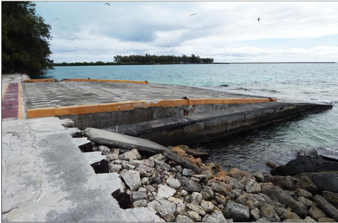
Figure 47: Seaplane Ramp (Property No. S2115), Midway Atoll, Sand Island (April 14, 2015)
