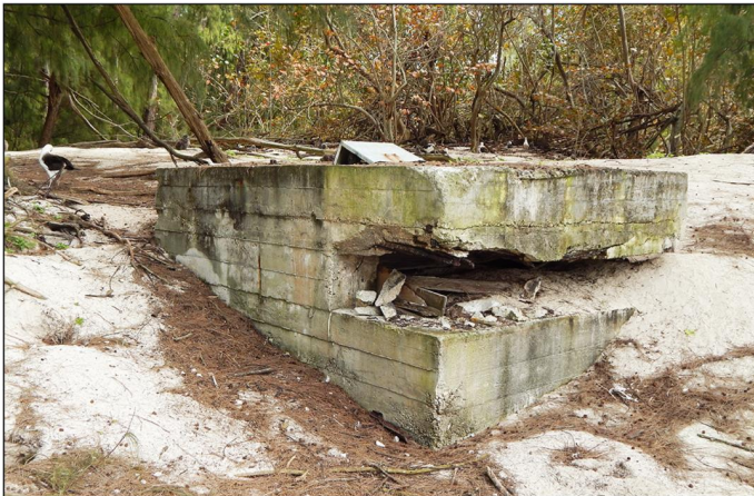
Figure 34: Concrete Pillbox (Property No. S-3), Midway Atoll, Sand Island (April 15, 2015)
