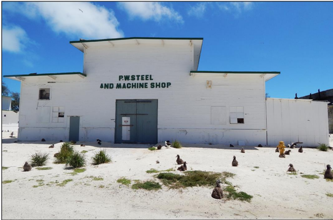
Figure 23: Torpedo Machine Shop (Property No. 357), Midway Atoll, Sand Island (April 13, 2015)
