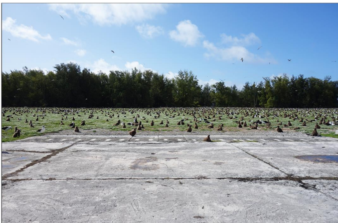
Figure 48: Seaplane Ramp (Property No. 2117), Midway Atoll, Sand Island (April 20, 2015)
