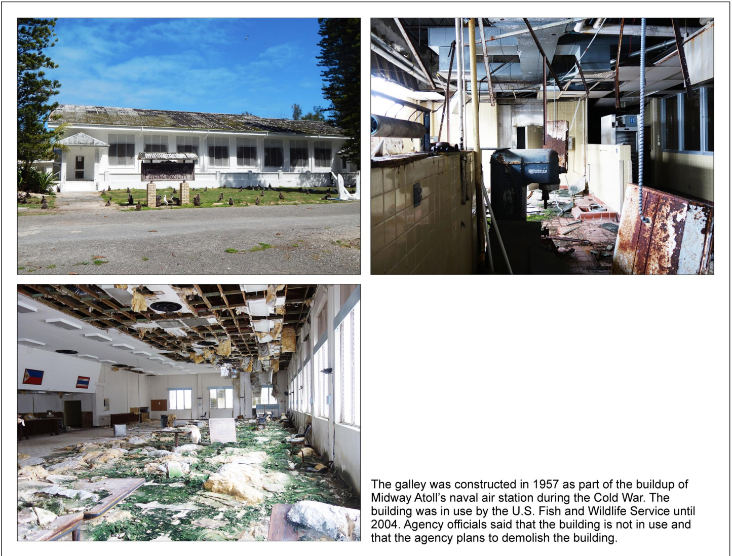
Figure 63: Galley (Property No. 3502), Midway Atoll, Sand Island (April 13, 2015, and April 17, 2015)
