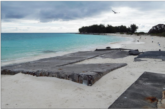
Figure 49: Seaplane Ramp (Property No. S9132), Midway Atoll, Sand Island (April 14, 2015)
