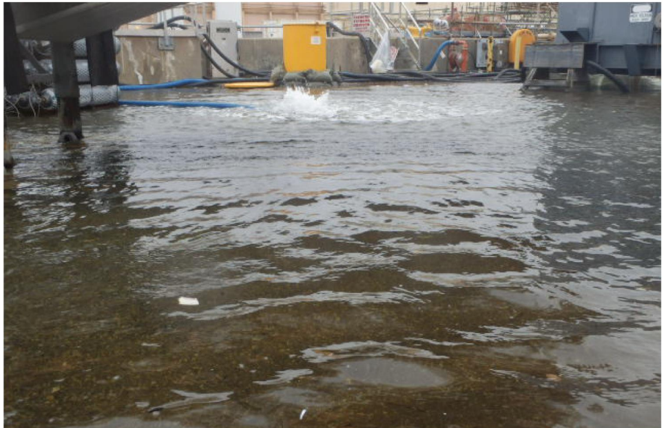
Figure 5: Flooding at Norfolk Naval Shipyard, Virginia
