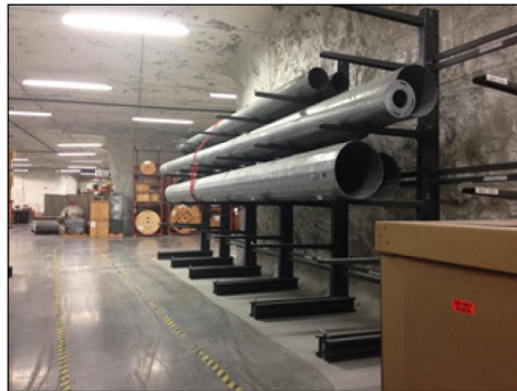
Components for wind shear alert system at the Staging Area in Independence, Missouri
