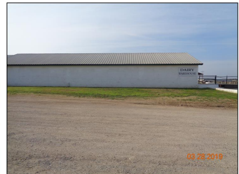
Exterior of a warehouse used to store dairy equipment and materials at Federal Correctional Institution El Reno
