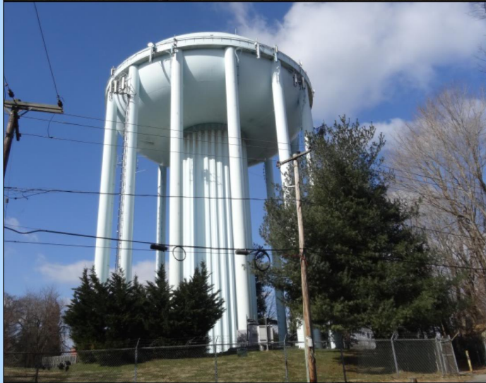
Water towers erroneously identified as leased office buildings by the General Services Administration in Laurel (top) and Bowie, Maryland.
