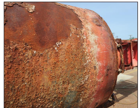
These 6' x 20' lighted steel buoys are eroded and rusty from extended periods of time in saltwater waterways, as well as continued exposure to other harsh maritime conditions.
