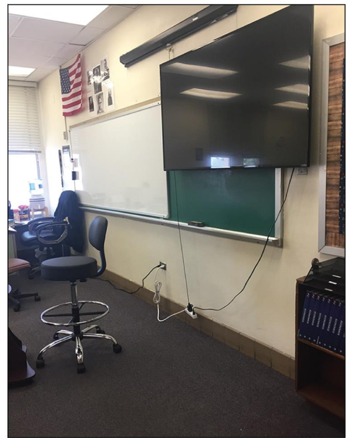
White board and screen placed on top of an old chalkboard so as to not disturb asbestos in the wall in a school in Florida.
