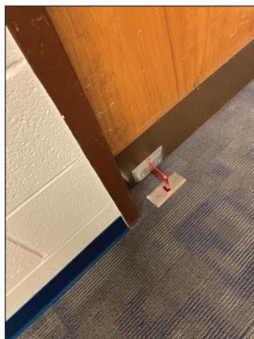
A supplemental barricade on a classroom door in a school in Michigan. Students are trained on how to use this in an emergency.
