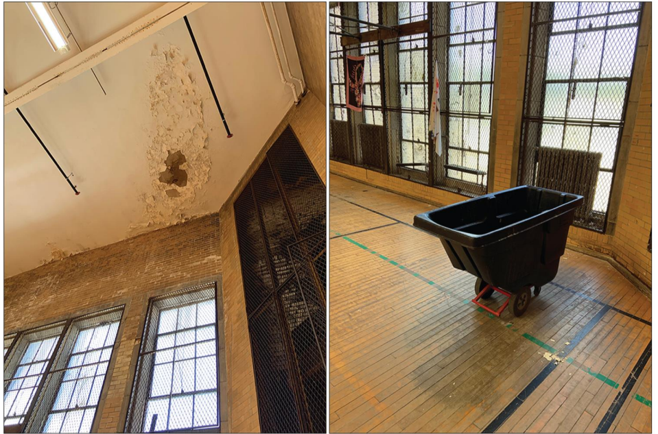
Roof leak in a Rhode Island school gym and bin underneath used to catch the water.
