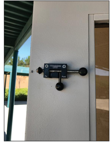
Door hardware that allows the door to be locked quickly in an emergency at a school in California.
