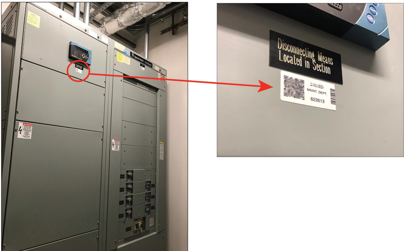
Figure 9: Barcodes Used to Help a California School District Track the Condition of Building Systems in its Public Schools
