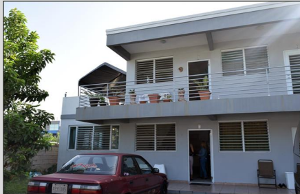
Source: GAO; photos taken by GAO while on site in Puerto Rico. | GAO-20-503
