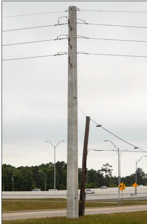
Figure 2. Wooden Utility Pole Replaced with a Concrete Pole
