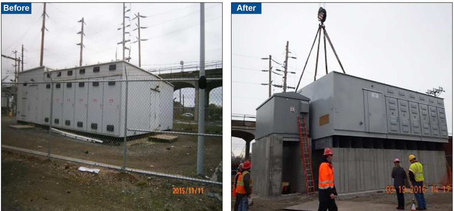
Figure 1: Elevated Substation in New York to Protect from Flooding
