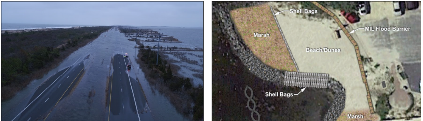
Figure 7: Flooding (Left) and Resilience Enhancements Made (Right) on Delaware State Route 1
