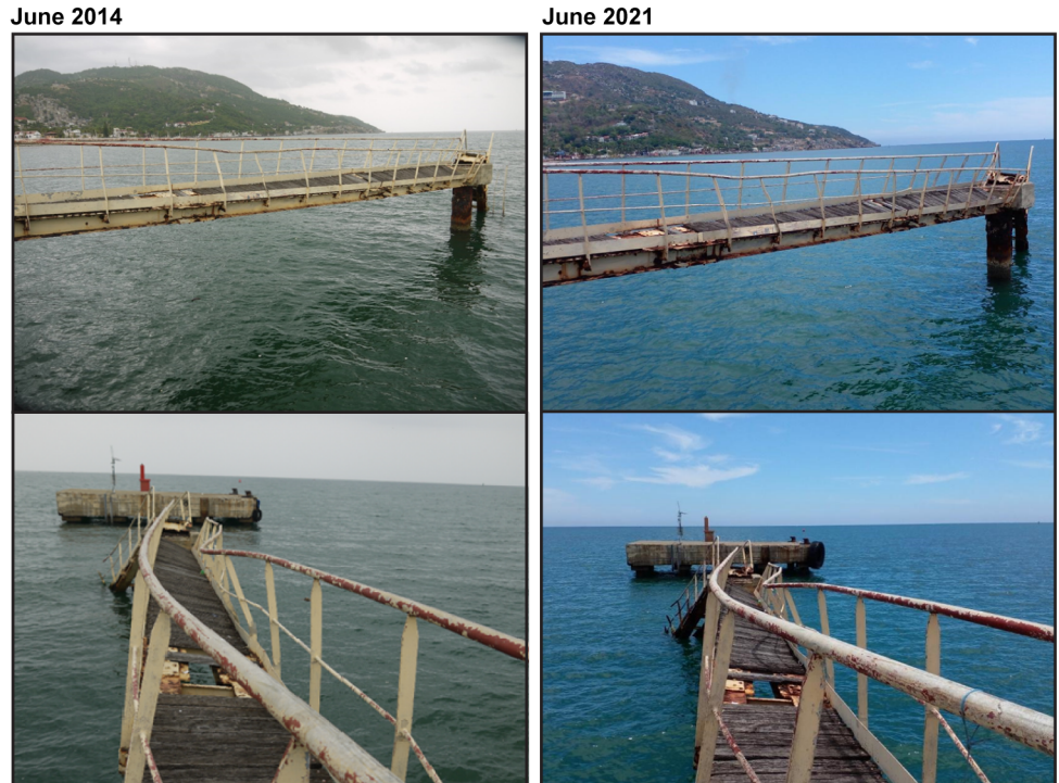
Figure 8: Comparison of Mooring Dolphins at the Cap-Haïtien Port in June 2014 (top left and bottom left) and in June 2021 (top right and bottom right) Showing No Change in Conditions Because USAID Reduced the Scope of its Port Renovation Activity
