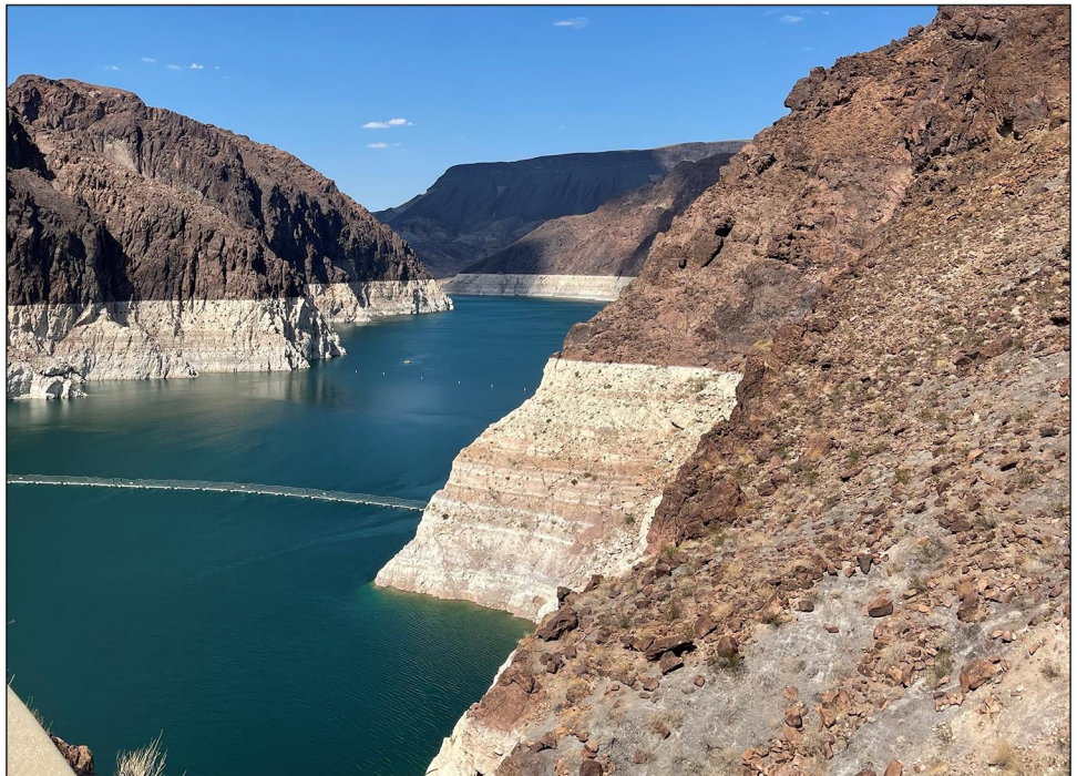
Figure 4: Low Water Levels at the Hoover Dam in August 2021
