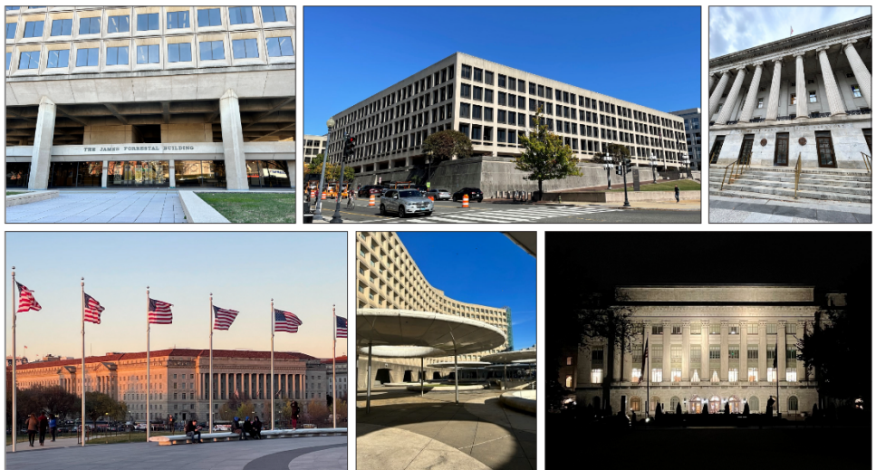
Figure 1: The Headquarters Buildings for the Departments of Energy, Labor, Treasury (top row), Commerce, Housing and Urban Development, and Agriculture (bottom row)
