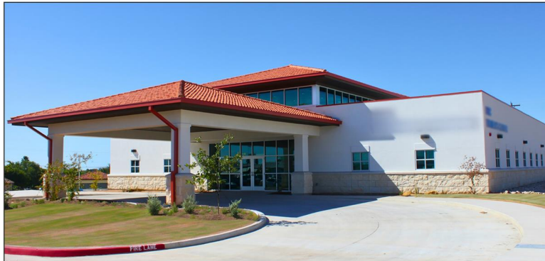
Figure 5: New Health Center Site Partly Funded by an American Rescue Plan Act of 2021 Capital and Construction Grant
