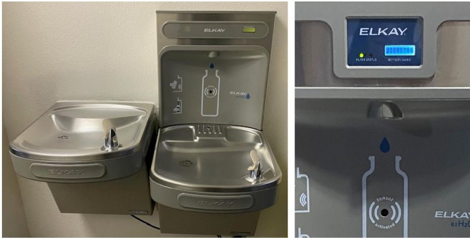
Figure 7: Water Bottler Refilling Station at a Department of Defense Installation and Total Plastic Bottles Avoided
