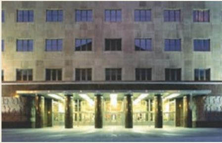
GAO headquarters building. Source: GAO Archives.
