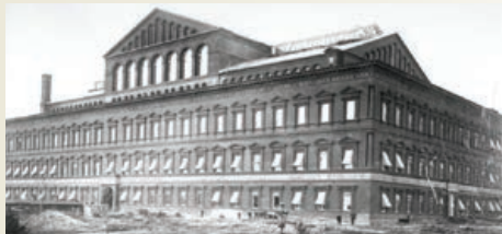
The Pension Building. Source: National Building Museum.
