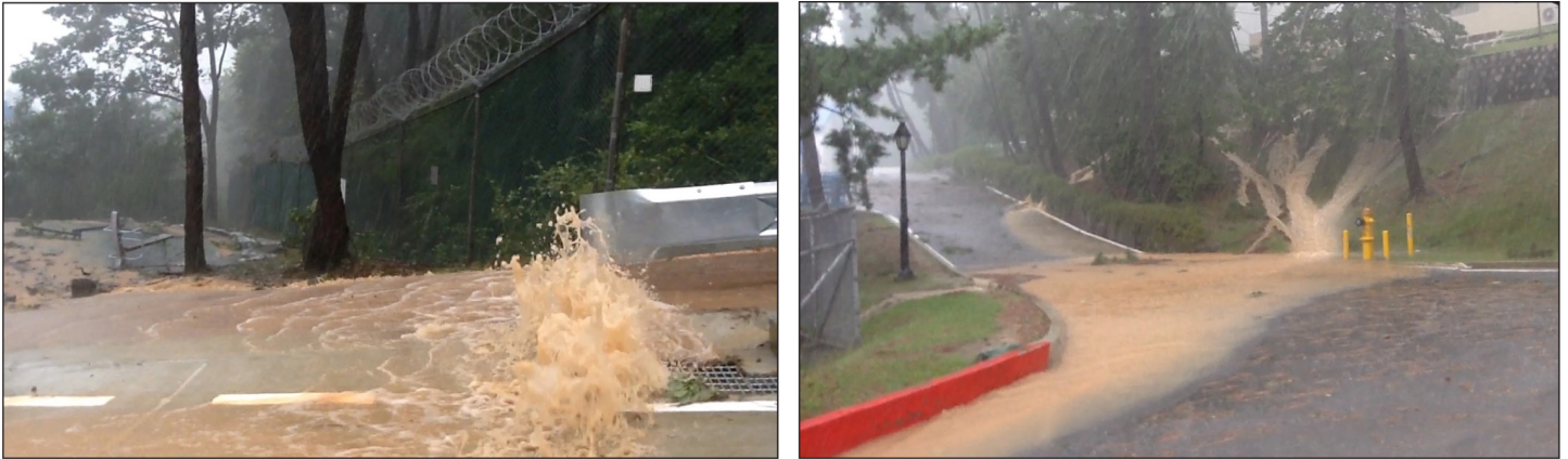
Figure 9: 2010 and 2014 Rainstorms Overwhelmed the Drainage System at a Department of Defense Installation in the Pacific
