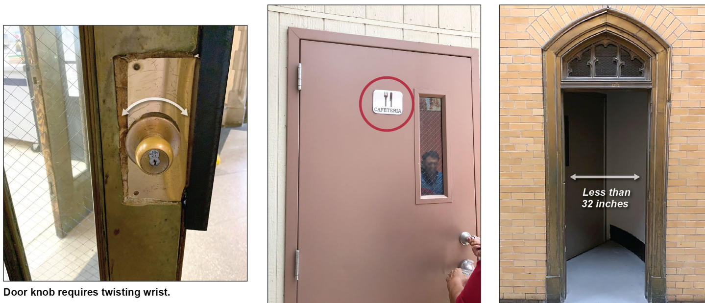
Sign located too high, located on door, and lacks raised characters or braille.
