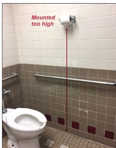
Toilet paper dispenser is placed at a high reach point.
