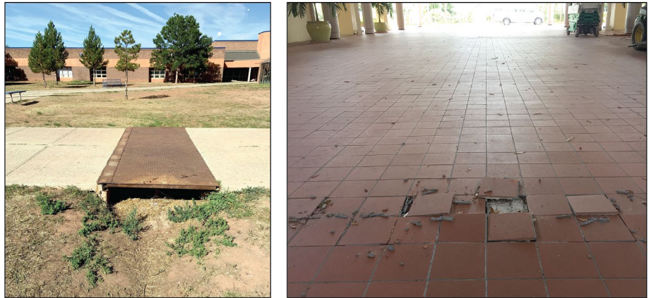
Uneven pathways (left) and large cracks in pathway surface (right).
