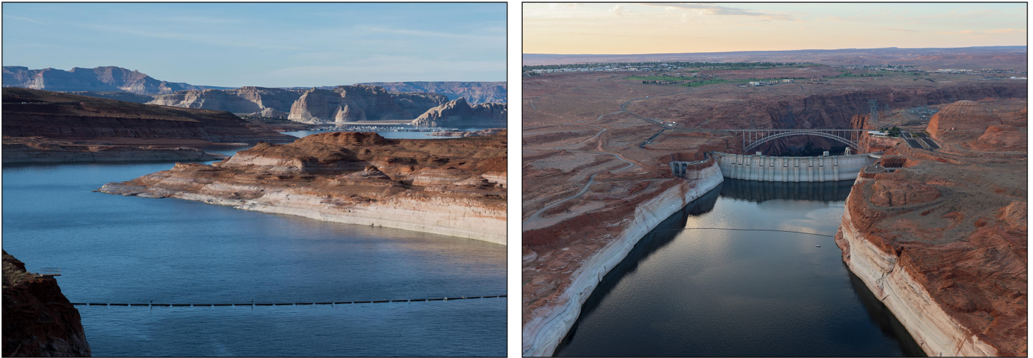
Figure 3: Low Water Levels at Lake Powell (left, 2017) and Glen Canyon Dam (right, 2021)
