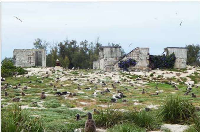
Figure 58: Small Radar Building (Property No. 631), Midway Atoll, Sand Island (April 14, 2015)
