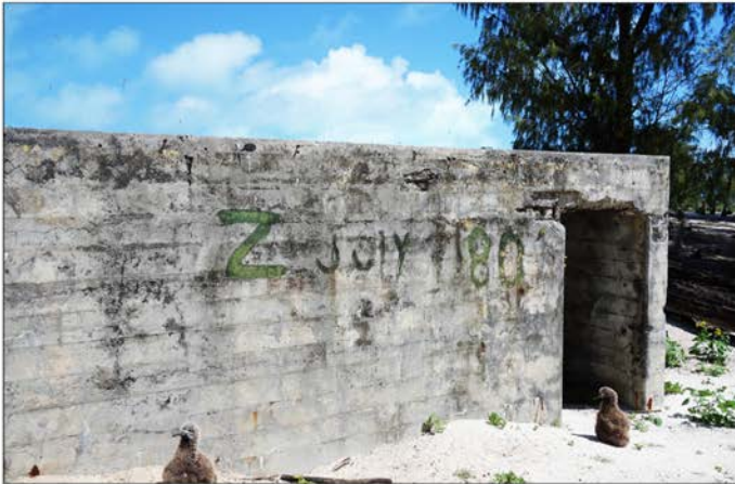
Figure 59: Radar Tower Bunker (Property No. 5187), Midway Atoll, Sand Island (April 20, 2015)
