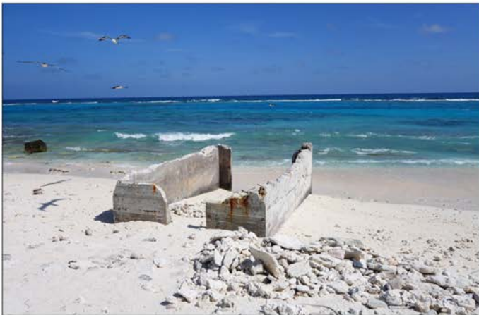
Figure 44: Underground Bunker (Property No. E-2), Midway Atoll, Eastern Island (April 16, 2015)
