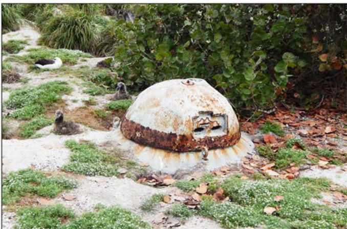
Figure 32: Metal Pillbox (Property No. S-7), Midway Atoll, Sand Island (April 14, 2015)
