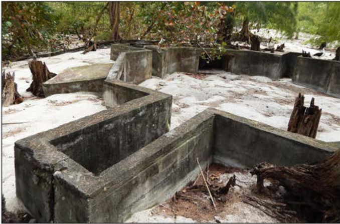
Figure 41: Battery D, 3-Inch Gun Position (Property No. S-2), Midway Atoll, Sand Island (April 15, 2015)
