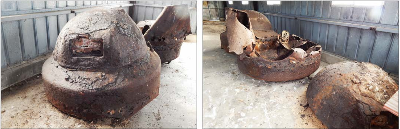
Figure 31: Metal Pillboxes (Property No. E-4), Midway Atoll, Sand Island (April 13, 2015)
