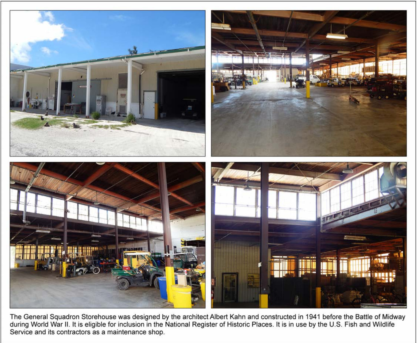
Figure 19: General Squadron Storehouse (Property No. 356), Midway Atoll, Sand Island (April 13, 2015)
