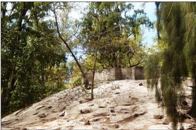
Figure 40: Battery C, 5-Inch Gun Position (Property No. S-1), Midway Atoll, Sand Island (April 14, 2015)
