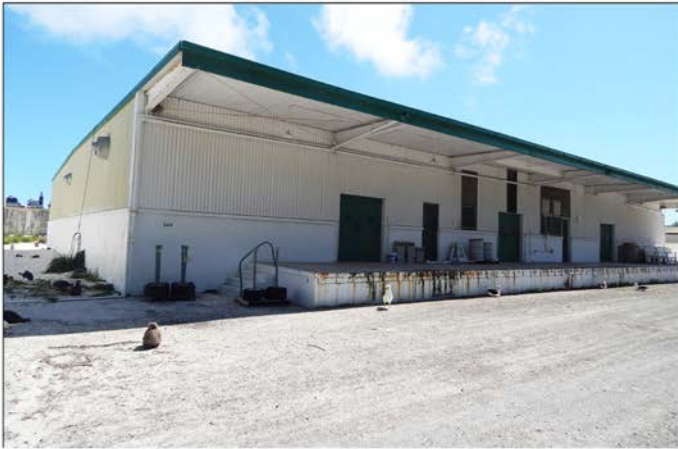
Figure 21: Commissary and Cold Storage (Property No. 349), Midway Atoll, Sand Island (April 13, 2015)
