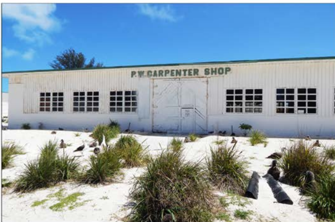
Figure 24: Carpentry Shop (Property No. 353), Midway Atoll, Sand Island (April 13, 2015)
