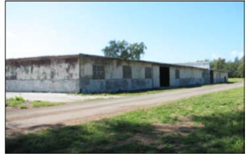
SK1 Warehouse (property number 393), 2007.
