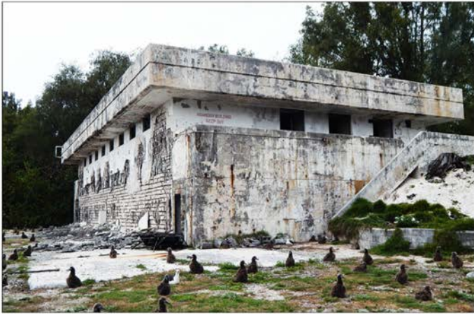
Figure 61: Command Post (Property No. 521), Midway Atoll, Sand Island (April 14, 2015)
