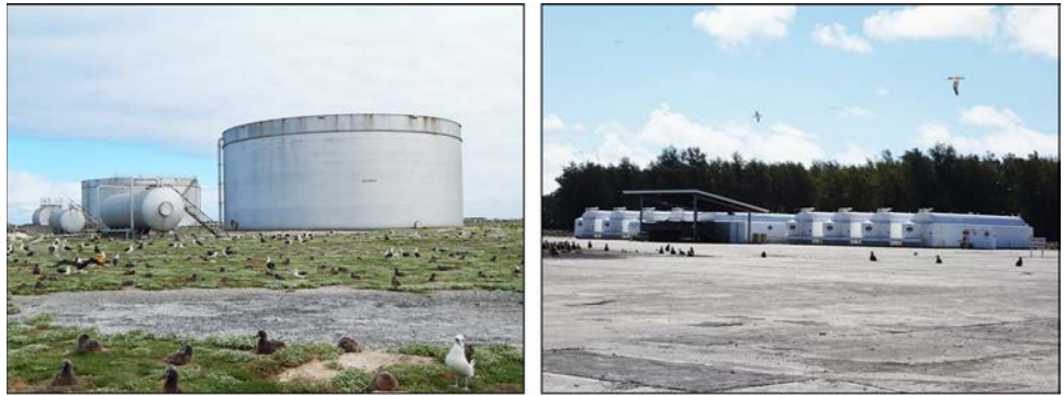
Figure 7: Photographs of Old Fuel System (Left) and New Fuel System (Right) on Midway Atoll, April 2015
