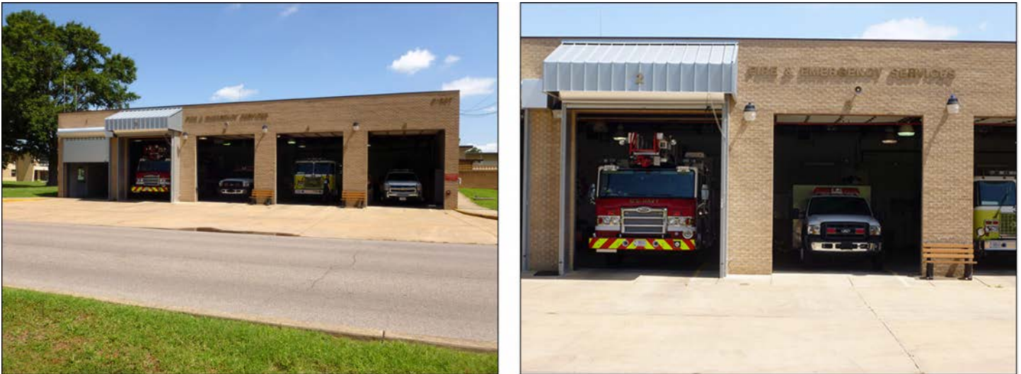
Figure 7: High Seismic Risk Unreinforced Masonry at Security and Fire Department Building on Navy Installation
