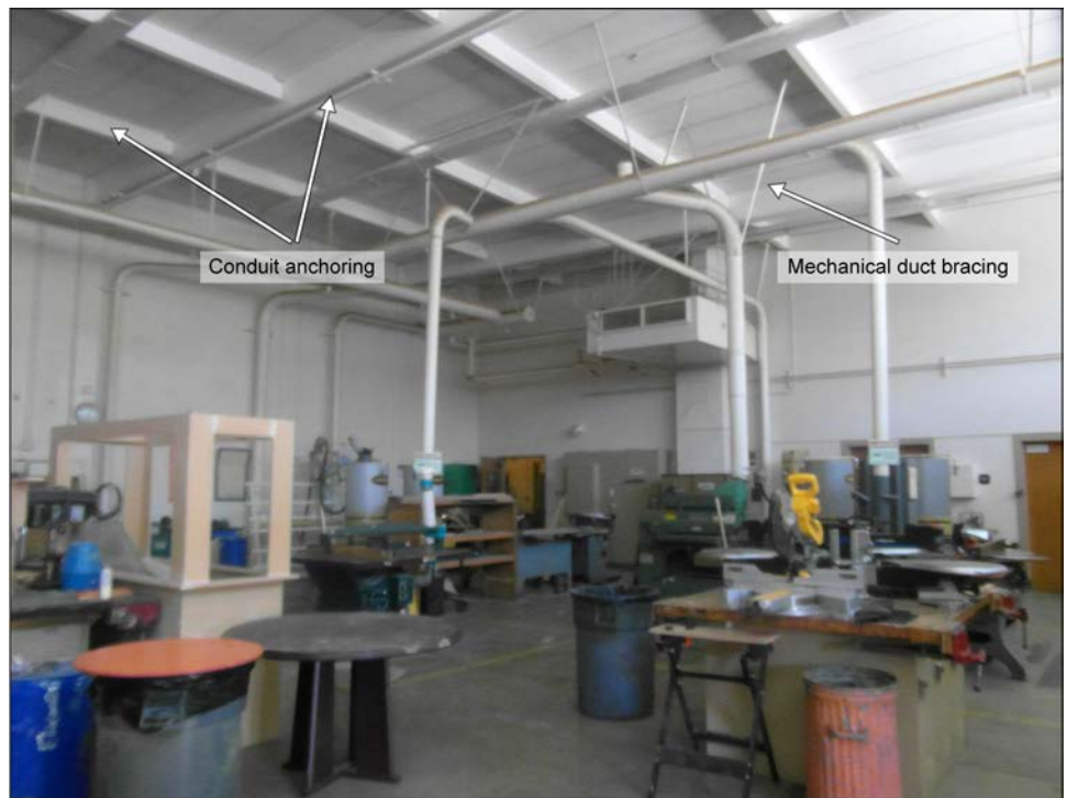
Figure 4: Anchoring and Bracing of Building Components in a Los Angeles Unified School District School Building
