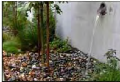
Downspout disconnection
