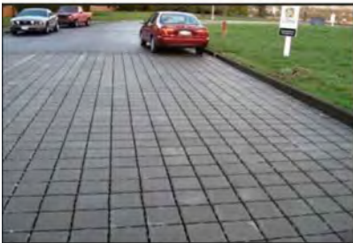
Permeable pavement
