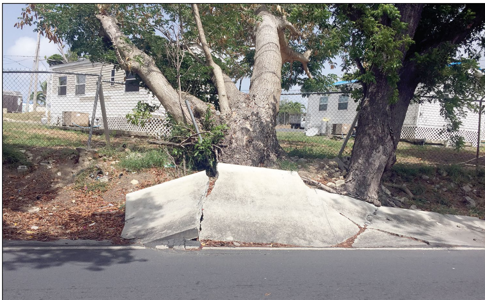
Figure 1: Storm Damage in St. Croix, the U.S. Virgin Islands
