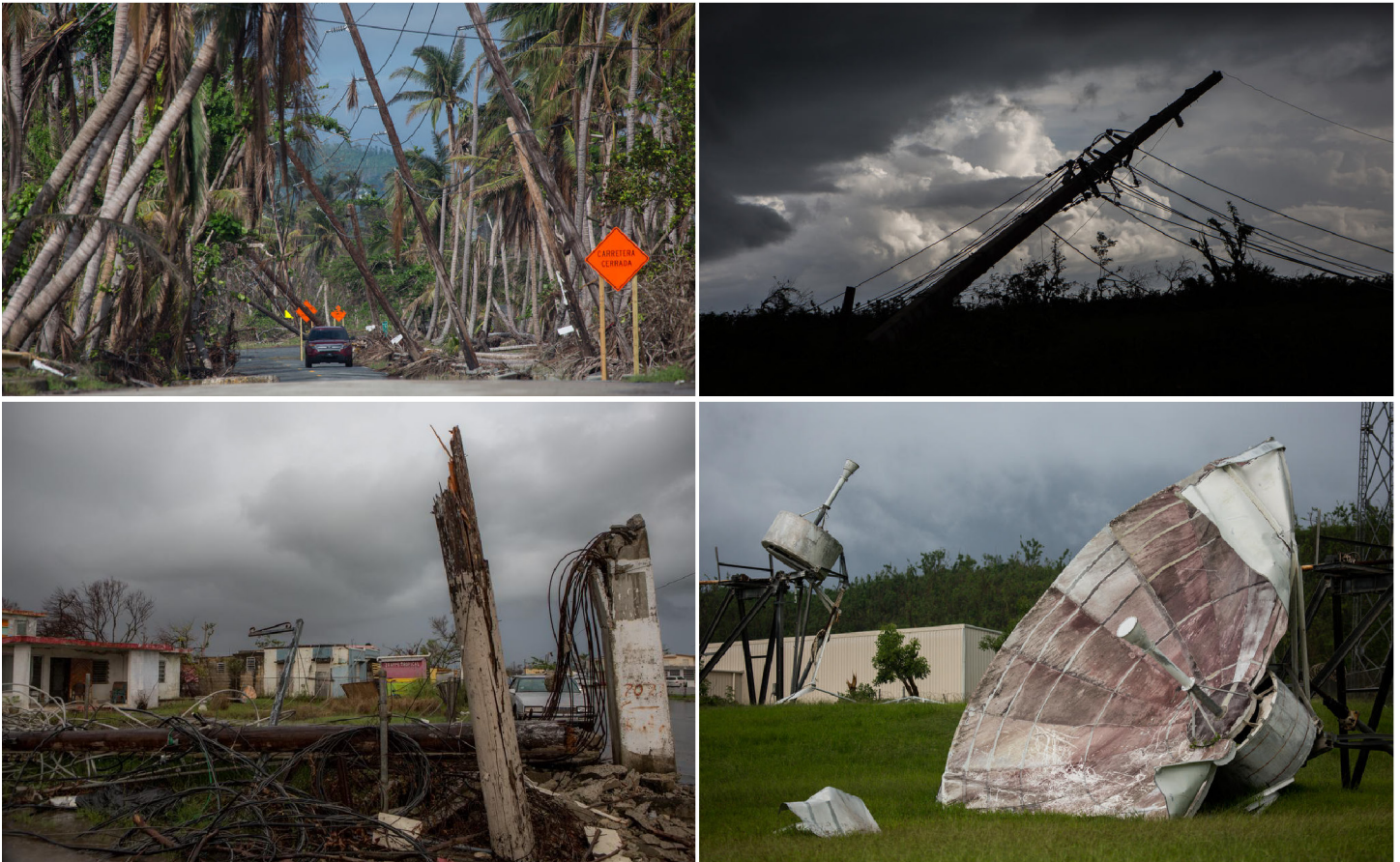
Figure 2: Damaged Power Lines and Satellite Dish in Puerto Rico after Hurricane Maria in November 2017
