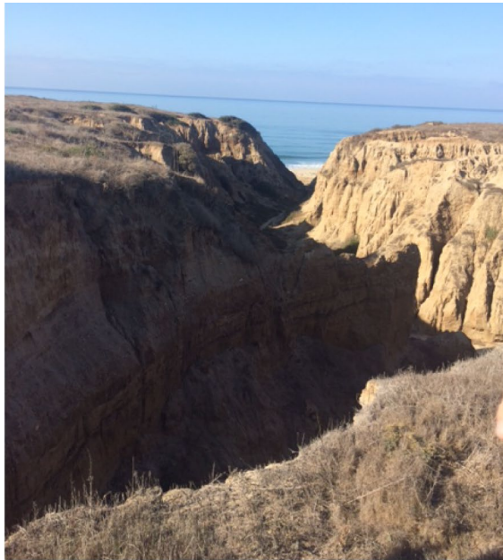
Figure 6: Coastal Erosion at Camp Pendleton, California
