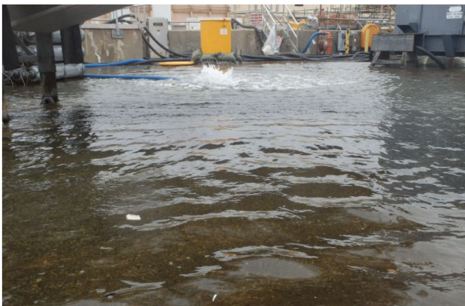
Figure 5: Flooding at Norfolk Naval Shipyard, Virginia
