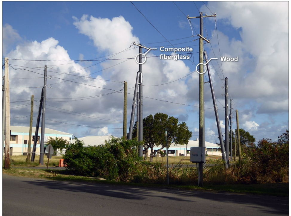
Figure 9: Wooden and New Composite Fiberglass Utility Poles in St. Croix, U.S. Virgin Islands
