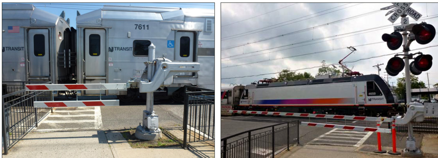
Figure 5: Photos of Gate Skirts for Pedestrians in Matawan, New Jersey
