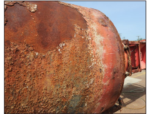
These 6' x 20' lighted steel buoys are eroded and rusty from extended periods of time in saltwater waterways, as well as continued exposure to other harsh maritime conditions.
