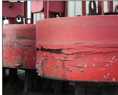
These 5' x 9' floating foam buoys are showing deterioration from continued exposure to harsh maritime conditions.
