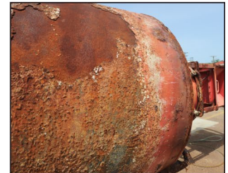
These 6' x 20' lighted steel buoys are eroded and rusty from extended exposure to saltwater and other harsh maritime conditions.
