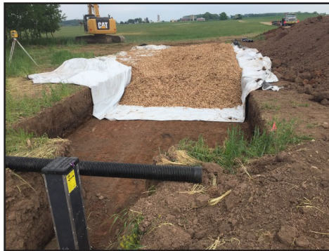
Bioreactor being filled with wood chips
