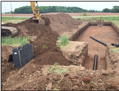
Bioreactor being built
