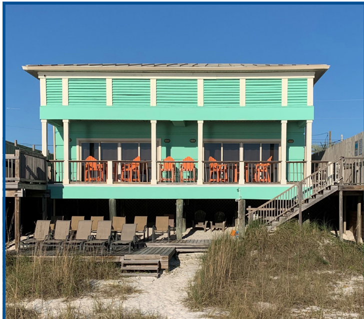
Structural elevation to mitigate flood damage, Panama City Beach, FL.
