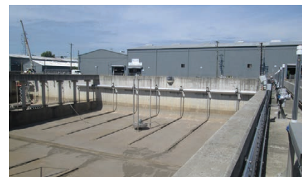
Driftwood Equalization Facility Improvement Project Source: Metro Water Services. | GAO-23-105285
