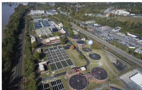
Capital Region Water's Advanced Wastewater Treatment Facility Source: Capital Region Water. | GAO-23-105285
