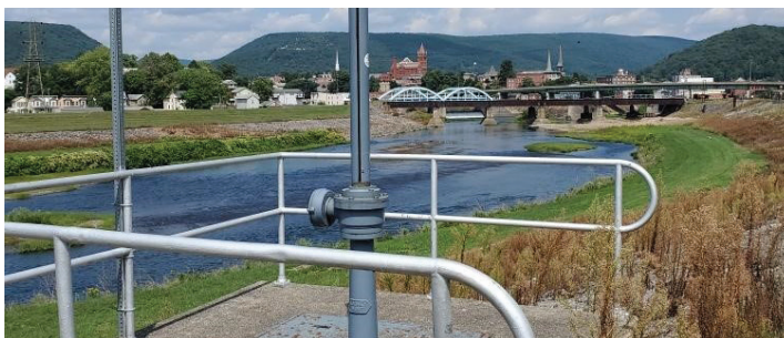
CSO outfall looking upstream at Potomac River, Cumberland, Maryland. Source: City of Cumberland, Maryland | GAO-23-105285
