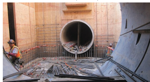
Construction of New Sunnydale Tunnel in 2011
