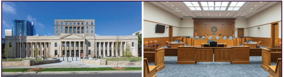
Exterior of Historic Jonas Federal Building (foreground) and New U.S. Courthouse Annex (background) (left), and Virginia Revival Courtroom Layout (right), Charlotte, NC
