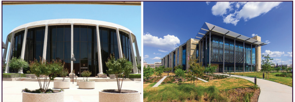
John H. Wood Jr. U.S. Courthouse (left) and New San Antonio Courthouse (right), San Antonio, TX
