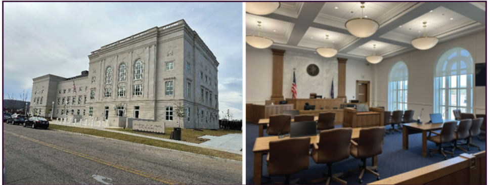
New Anniston Courthouse (left) and Courtroom with Windows to Maximize Natural Light (right), Anniston, AL
