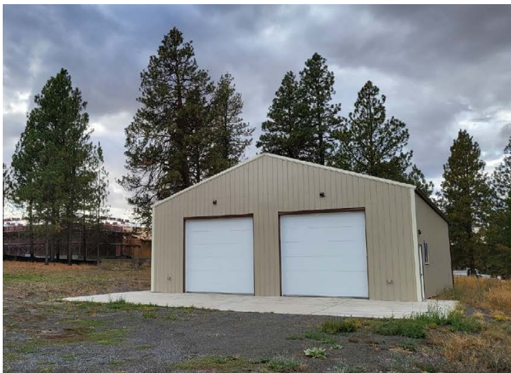
Temporary fire station
