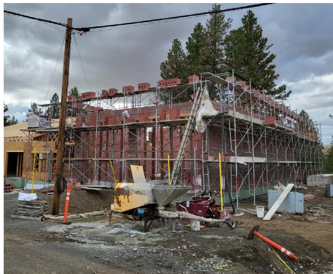
Construction on town hall
