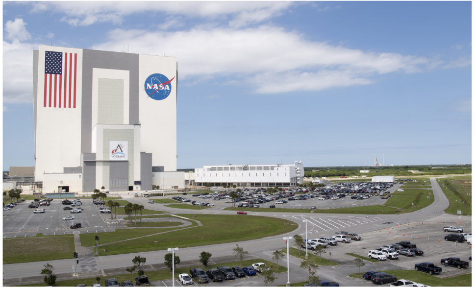
Figure 3: Photo of the Vehicle Assembly Building
