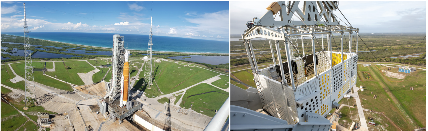
Figure 2: Photos of Launch Pad 39B and the Emergency Egress System
