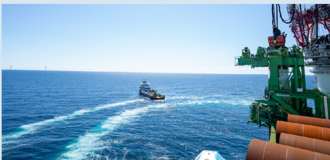
Double bubble curtain surrounding pile driving operations at an offshore wind site.
